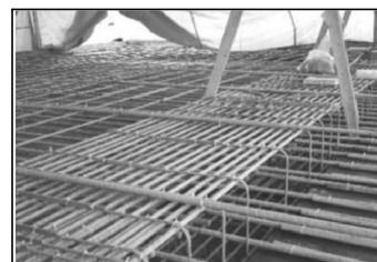
Figura 7. Barre e staffe in GFRP
