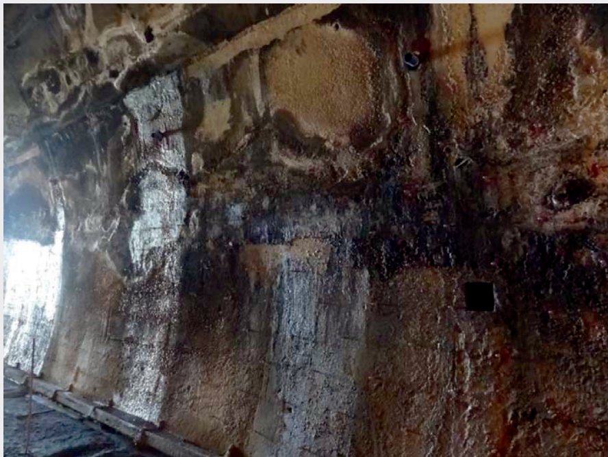
Fig. 10. Fessure diffuse, bagnate
