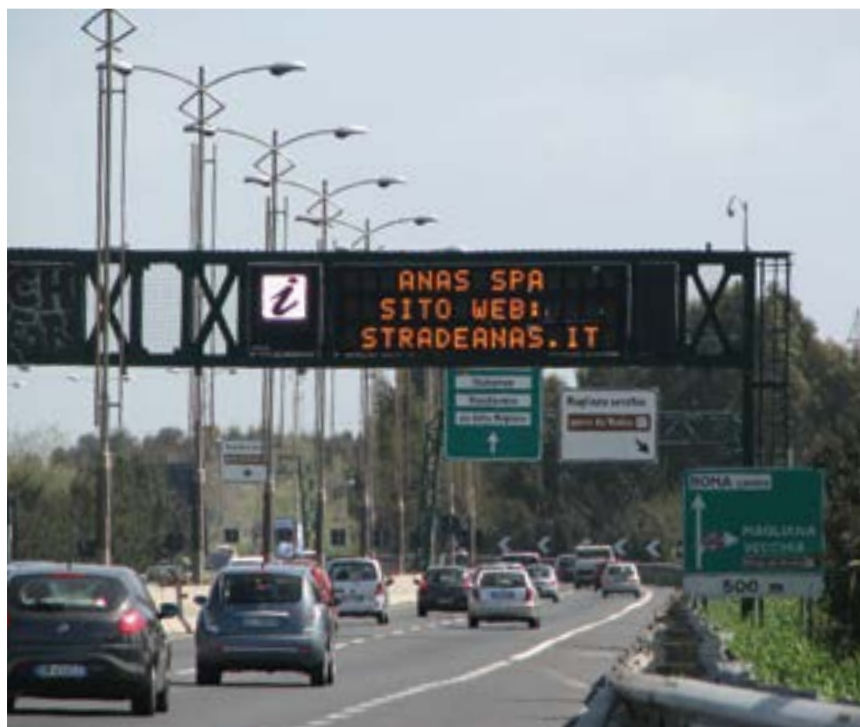
G.R.A. Highway of Rome - Variable message signs
