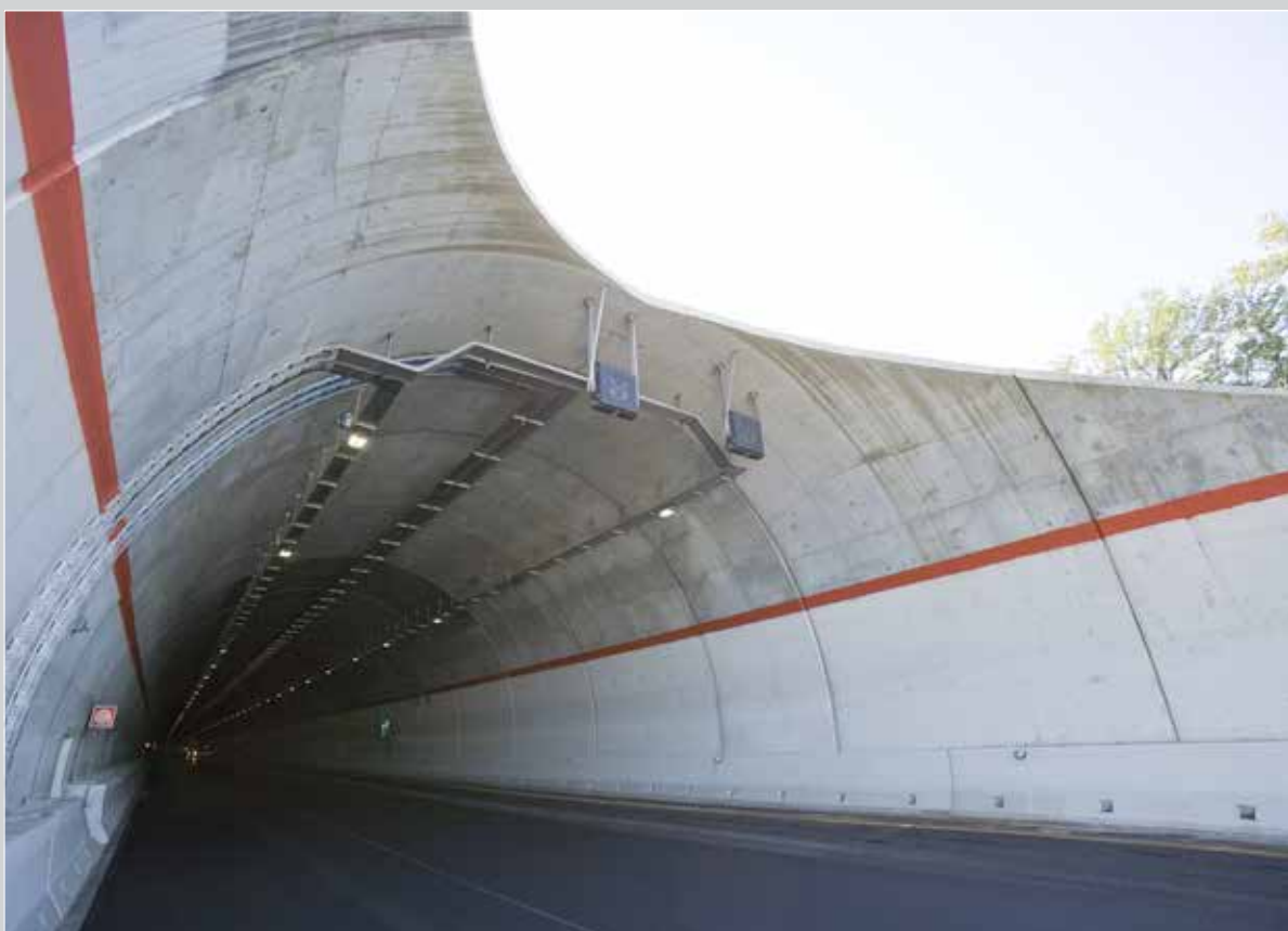
■ Motorway A3 Salerno-Reggio Calabria - Gallery North Cerreta
