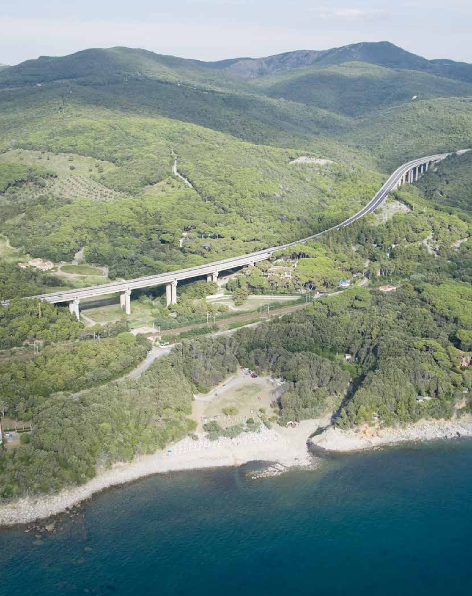
■ S.S. 1 "Aurelia" - Location Fortullino Two Viaducts
